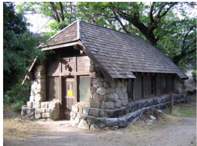
A Yosemite restroom, built by the CCC.
